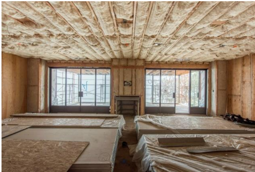
Figure 5. Sheep's wool is incorporated into the ceiling
